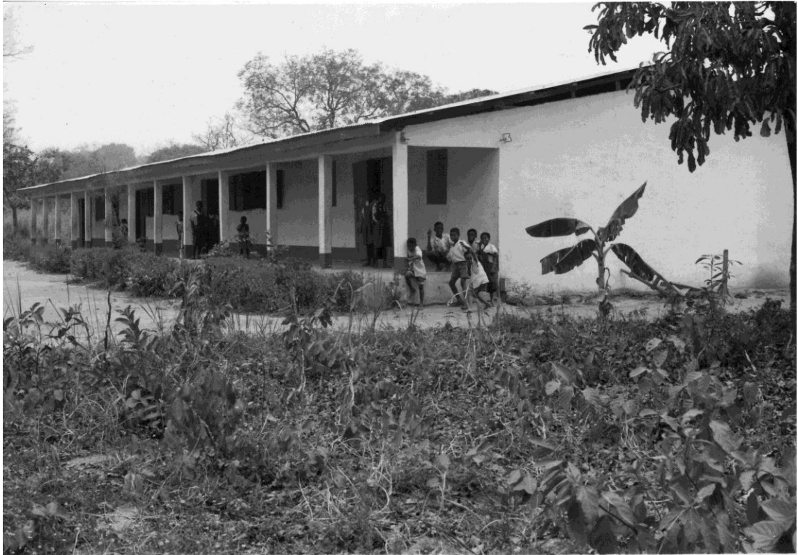
PRIMARY SCHOOL BLOCK CONSTRUCTED BY WORLD VISION AT SAMARI-NKWANTA
