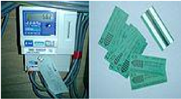
Figure 4.0. A magnetic/token prepayment system
